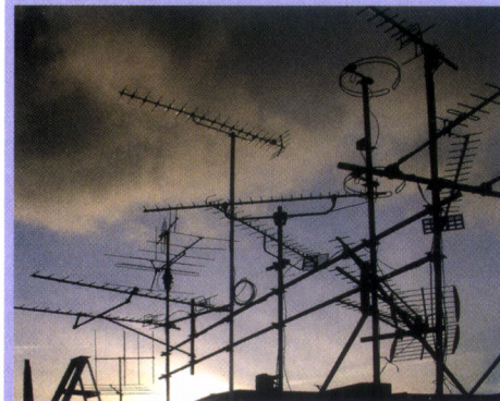
After analogue switch off the increased power of the digital signals will make many big aerials like these unnecessary
